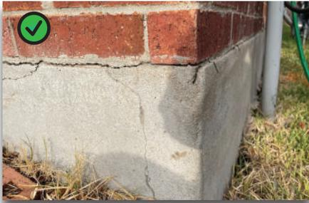
Typically there is a cosmetic skim coating applied to the exterior of the foundation once the forms come off. Cracks can develop there for multiple reasons without there being an actual issue with the foundation.
