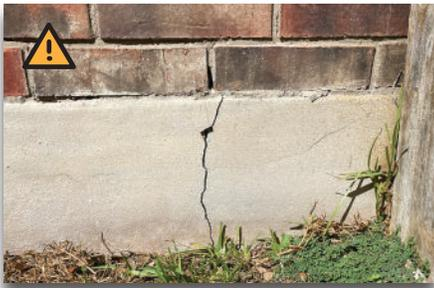
Cracks in the foundation that have separation and are deeper than the skim coat can be a sign of a more serious issue.
