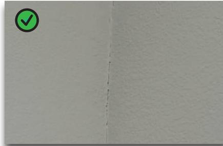
Hairline cracks, especially ones at tape seams, are signs of typical movement. Several factors can cause drywall cracks, such as changes in humidity, condition of framing, consistency of joint compound, etc.
