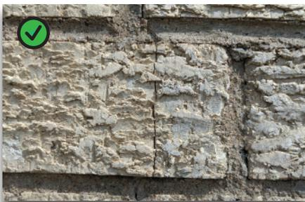
Hairline cracks through the middle of the rocks or bricks are signs of typical settlement or changes from moisture and temperature.
