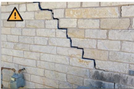
Stair-step cracks through the mortar with separation can be a sign of a potential deflection in the foundation and warrant further investigation.
