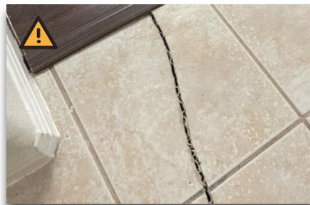
Cracks that run through multiple tiles in a straight line (especially with separation) could be a sign that something needs to be addressed.
