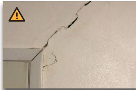
However, diagonal cracks with separation, especially at windows and door frames, can be a sign of foundation movement and could need additional evaluation.
