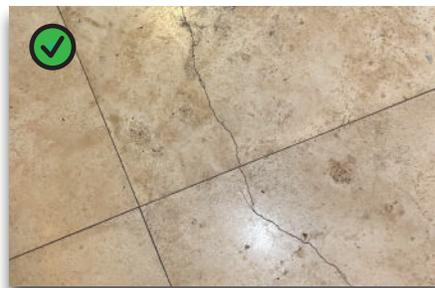
Hairline cracks in individual tiles are somewhat common and are not indicative of an issue with the foundation. There could be issues with the bond adhesion or the underlayment.
